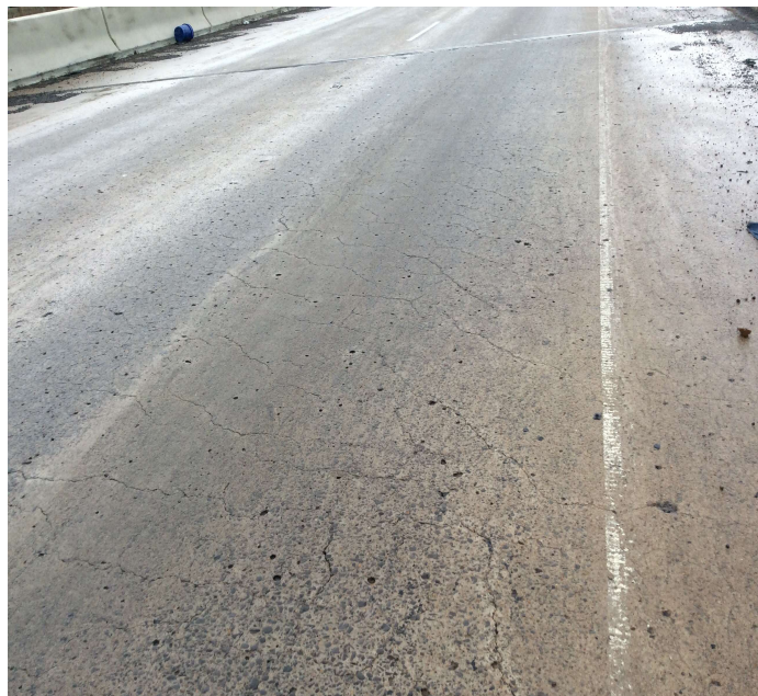
PHOTO 1 Description Span # 1 Heavy map cracking in the driving surface
