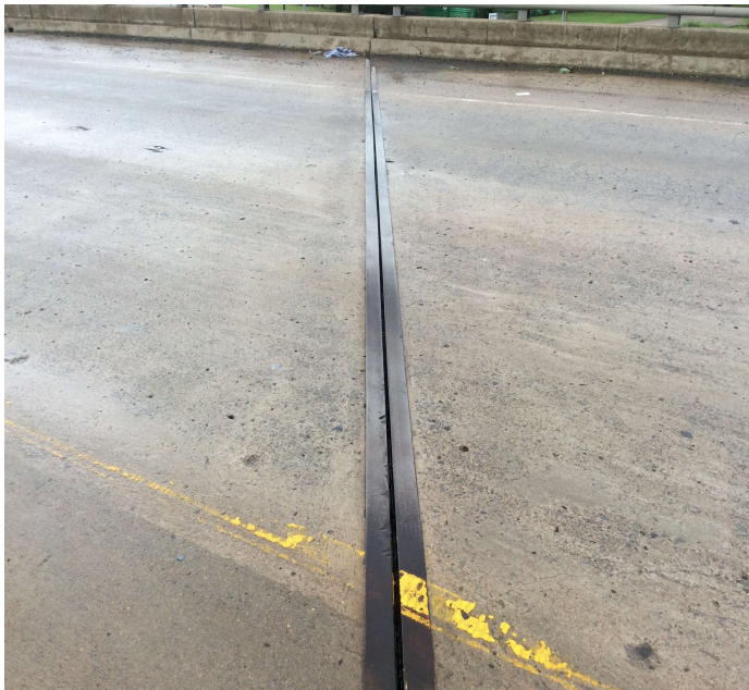
PHOTO 1 Description Bent # 3 missing joint seal
