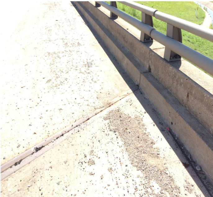
PHOTO 3 Description Expansion joint over Bent 3. Fully closed with a 1/4" elevation difference in the Right gutter.
