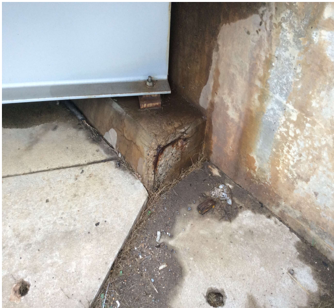
PHOTO 1 Description Bent # 4 Bridge seat spalling with exposed reinforcing steel
