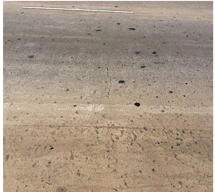
PHOTO 6 Description Sealable deck cracks Span 3
