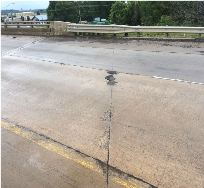
PHOTO 1 Description Bent # 1 Approach slab scaling with repairs
