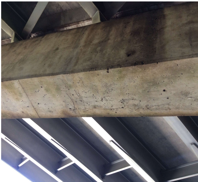
PHOTO 4 Description Delaminated areas under Bent 3 cap.
