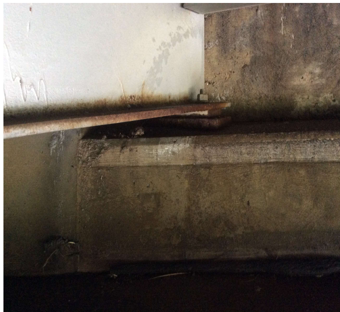
PHOTO 1 Description Bent # 4 Beam # 2 Active corrosion in the bearings
