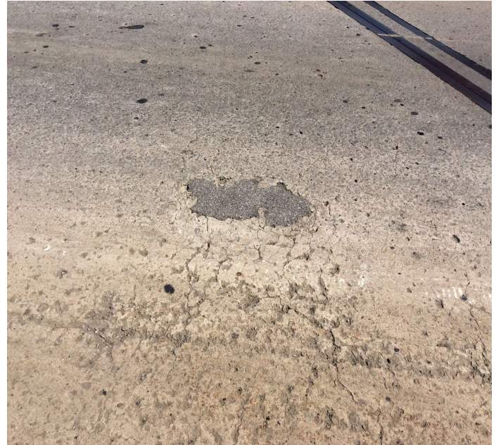
PHOTO 5 Description Spall with asphalt patch in Span 3.
