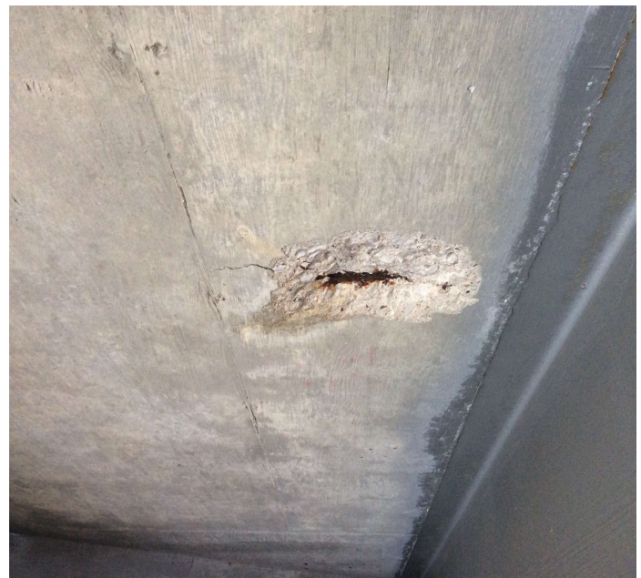
PHOTO 2 Description Span # 1 Bay # 6 Spalling with exposed reinforcing steel in the undersurface.
