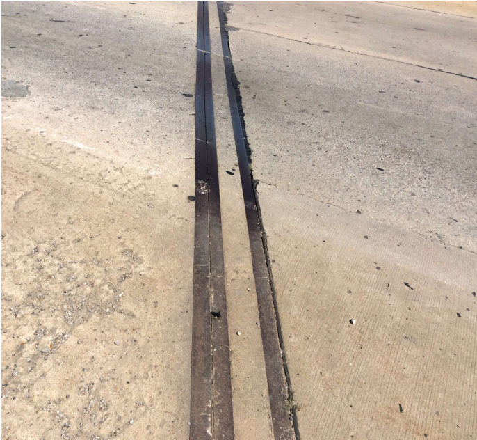
PHOTO 3 Description Expansion joint at Bent 4.
